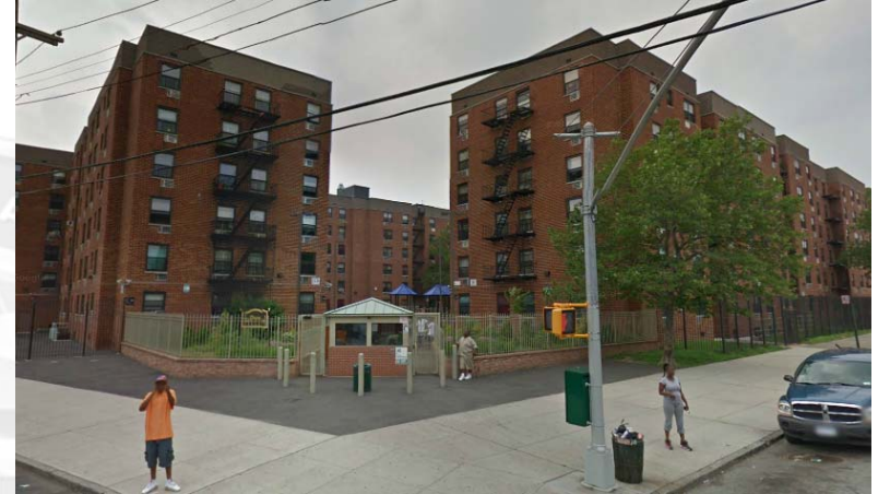
Noble Drew Ali apartment complex. [source: Google Maps, June 2011 image].
